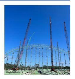
Additionally, Zamil Steel Vietnam is constructing a coal shed for a prestigious customer in Indonesia. The project weighs 2,300 metric tons and features steel arch trusses with a clear span of 130 meters using hollow sections. The welding and fabrication work for this project must meet extremely high standards.
