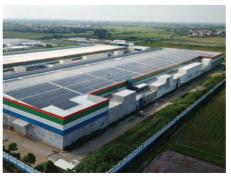
Located in Thai Binh Province in northern Vietnam, the factory covers a built-up area of 28,650 square meters. It features a clear span of 60 meters and uses multicolored sandwich panels for the walls.
