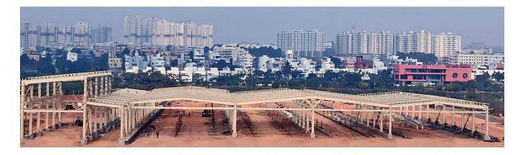
Zamil Steel Buildings India, through Parnika Commercial and Estates Pvt. Ltd., is constructing a metro depot for Bengaluru Metro Rail Corporation (BMRCL) in Bangalore. The scope of work includes the design, manufacture, supply, and erection of pre-engineered steel buildings for the metro depot, which covers an area of 22,000 square meters.
