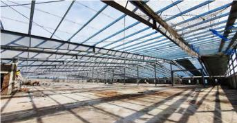
side – were used to create unobstructed spaces for various functions while still maintaining structural rigidity. The building was also equipped with the MaxSEAM® roof system for better weather resistance.
