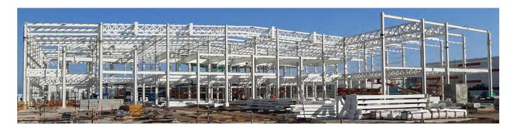
Zamil Steel Buildings India has recently been selected by a European Pharmaceutical Company to set up its production facility in Maharashtra state in western India. The scope of the contract includes the design, detail, manufacture, supply, and erection of more than 16,350 square meters of structural steel buildings, as well as relevant substructures and accessories.
