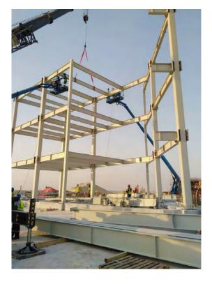
in the time it will take to erect the steel. Zamil Industrial brought this new American modular system to the Kingdom of Saudi Arabia, and the company has a specialized factory in Dammam to produce steel structures using the ConXtech system.
