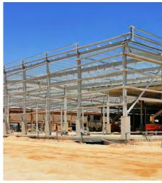
Zamil Steel has successfully completed the contract awarded by Al Bawani Company for the supply and erection of pre-engineered steel buildings for a new Saudia Cargo terminal in Riyadh, Saudi Arabia.
